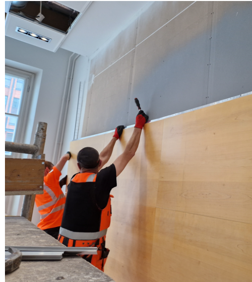
Figure 18. Deconstruction workers removing the veneer wood panel as instructed in the deconstruction instructions.
