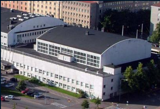
Töölö Sports Hall Rebar structure, beam localisation
