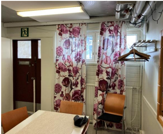
South Façade Window
